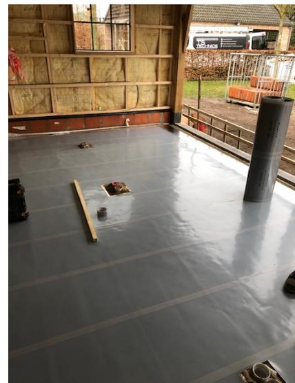
Compared to other electric heating systems, the energy from heating film converts into infrared rays without any energy waste. It consists of two copper strips, which works as the electrical power conductor. Due to its parallel structure our heating film lets you to heat the whole house efficiently and evenly.
