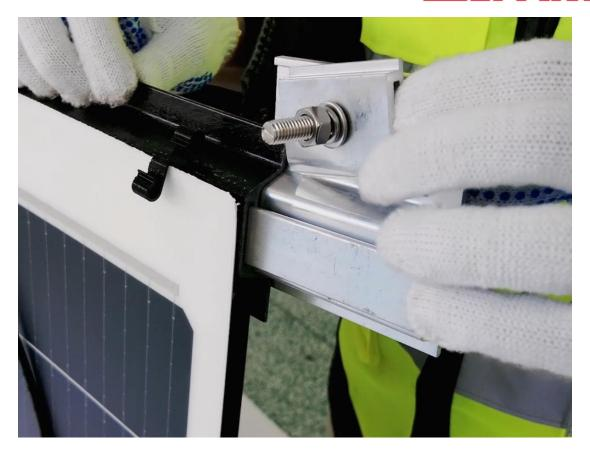
■ Place the modules with prefabricated units on the base.
